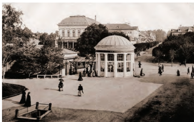
The spa centre, looking toward Franz’s Spring and the Kurhaus, 1898
