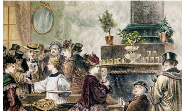
In the pump room
