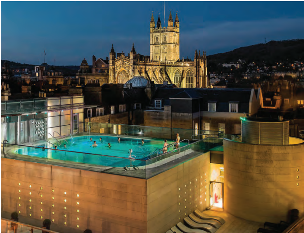
Thermae Bath Spa has sustained the continuing spa function of the City of Bath and was completed in 2003
